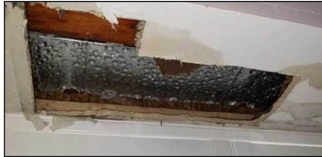
Damage caused by sweating ducts
